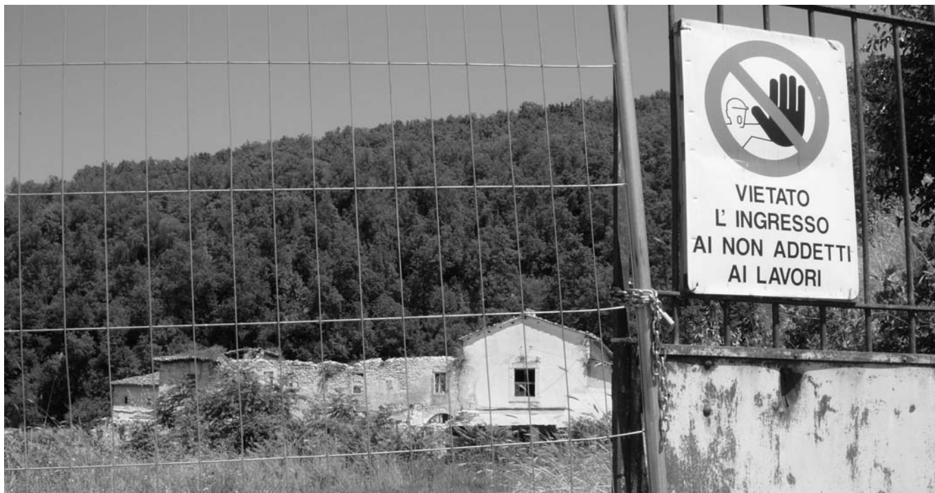
The Project on hold. The sign says: “Entry prohibited except for authorized workers”
