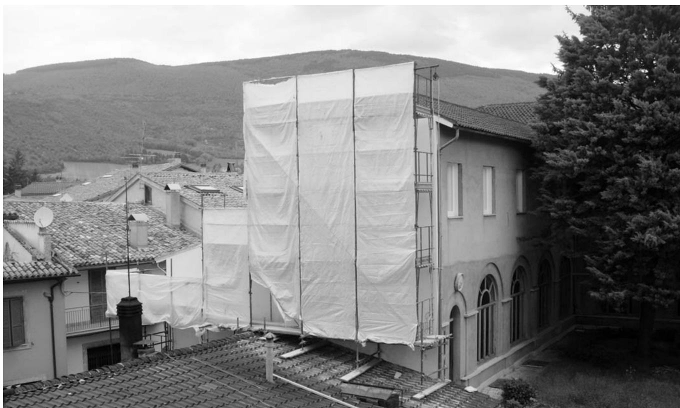
Scaffolding covers the noviate roof during repairs.
